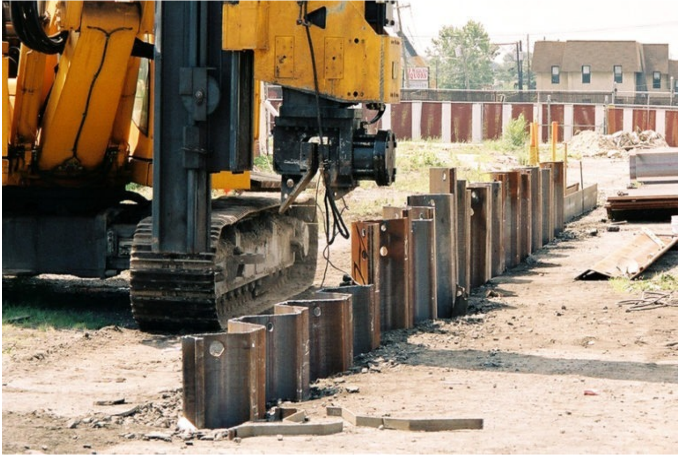
Sheet pile installation
