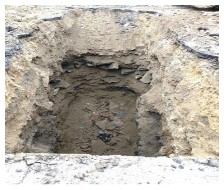
If your test borings show small amounts of brick, wood, or concrete, you might think you're dealing with common urban fill. But, then, surprise! Construction starts, and you find that the fill contains a significant amount of building rubble debris, which makes your contractor fear asbestos.
