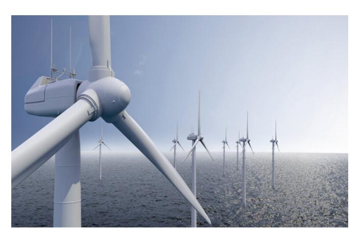
Environmental loading from wind and waves is highly uncertain. Design codes and guidelines help engineers predict the loads that an offshore wind turbine must resist during the design life of the structure, but these loads are estimated using statistical methods based on historical data. The U.S. East Coast experiences annual hurricanes, and
