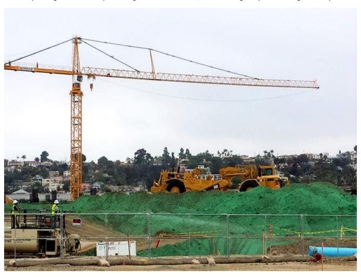
Inactive soil stockpiles were sprayed with bonded fiber matrix to provide stabilization during the rainy season.
