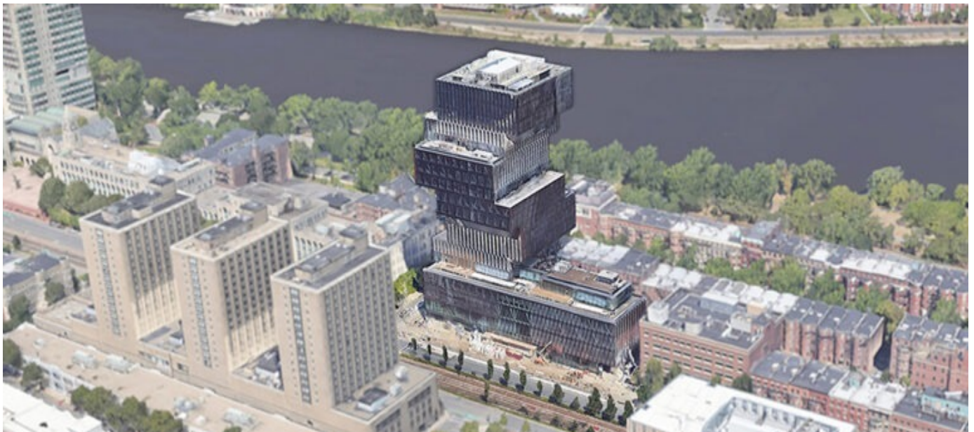
Boston University Center for Computing and Data Services (BUCCDS) building
