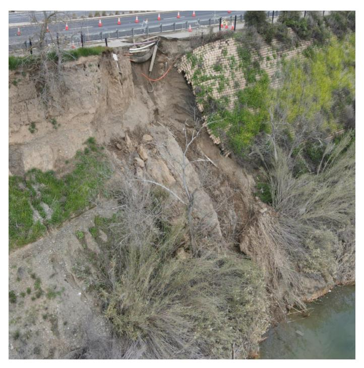
Two examples of geohazards that resulted from severe storm systems in the San Francisco Bay area in early 2023. An overwhelmed San Leandro Creek caused an embankment failure beneath A Street in Hayward (left). What started as a sinkhole developed into an embankment failure in Pleasanton (right).—
